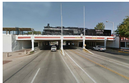
Figure 70: Douglas Avenue Underpass
