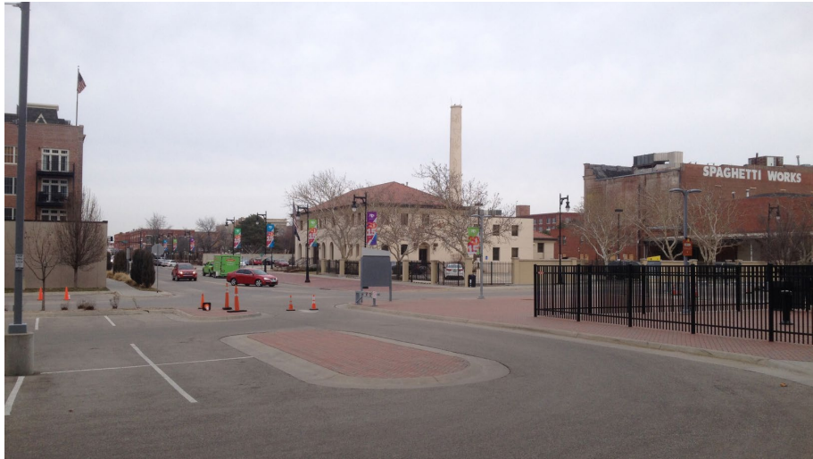
Figure 94: Existing Street View Exiting Intrust Bank Arena
