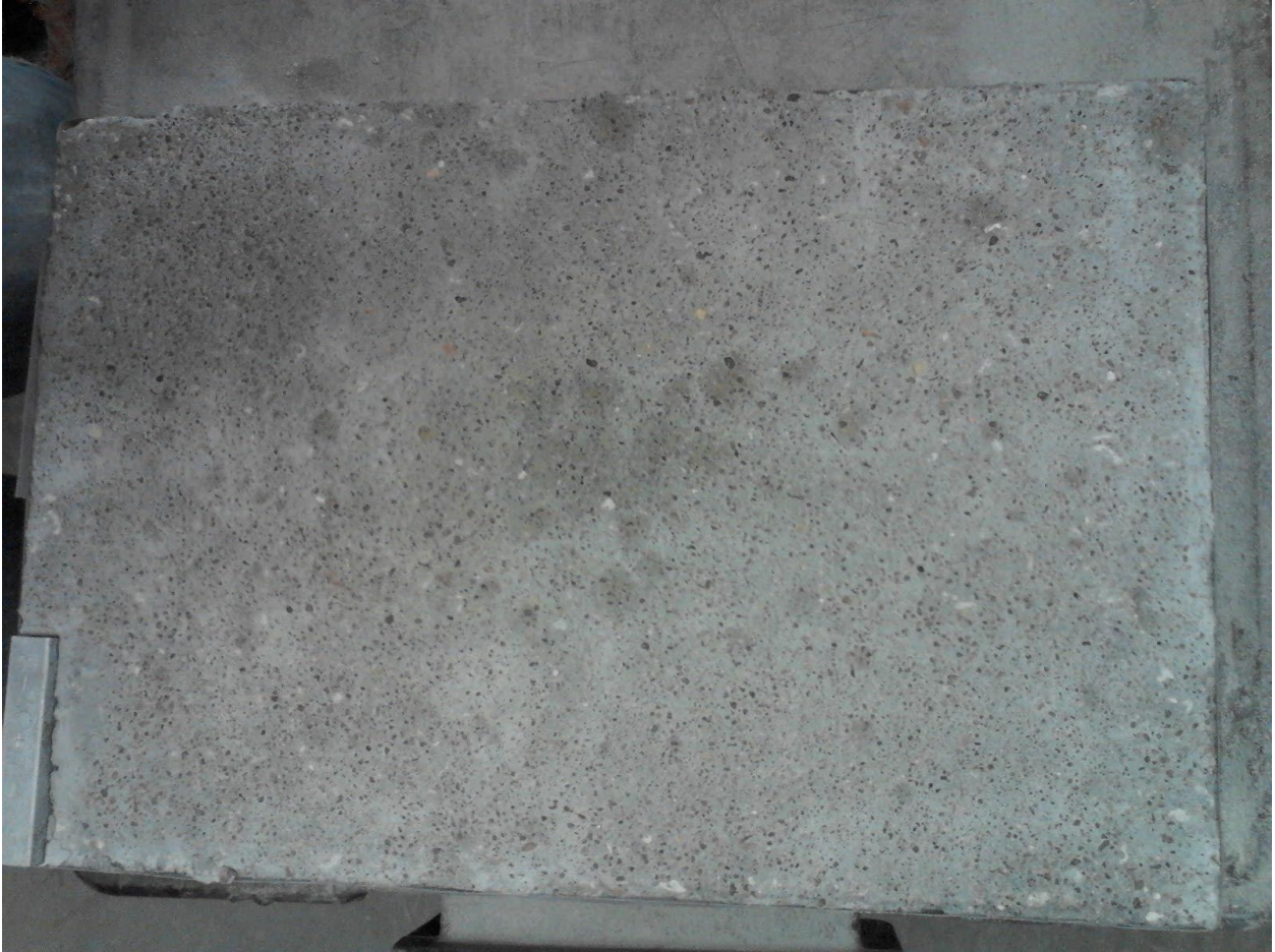
Figure 17: Sand blasted surface with visible large aggregates
