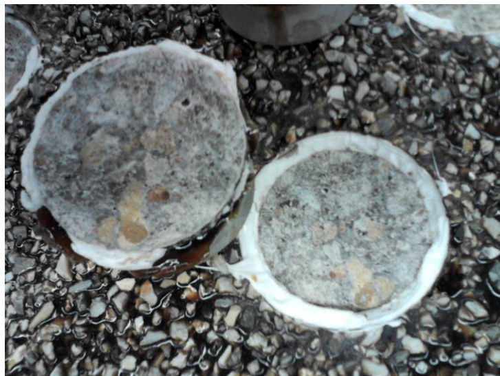
Figure 1: Failures in the concrete
