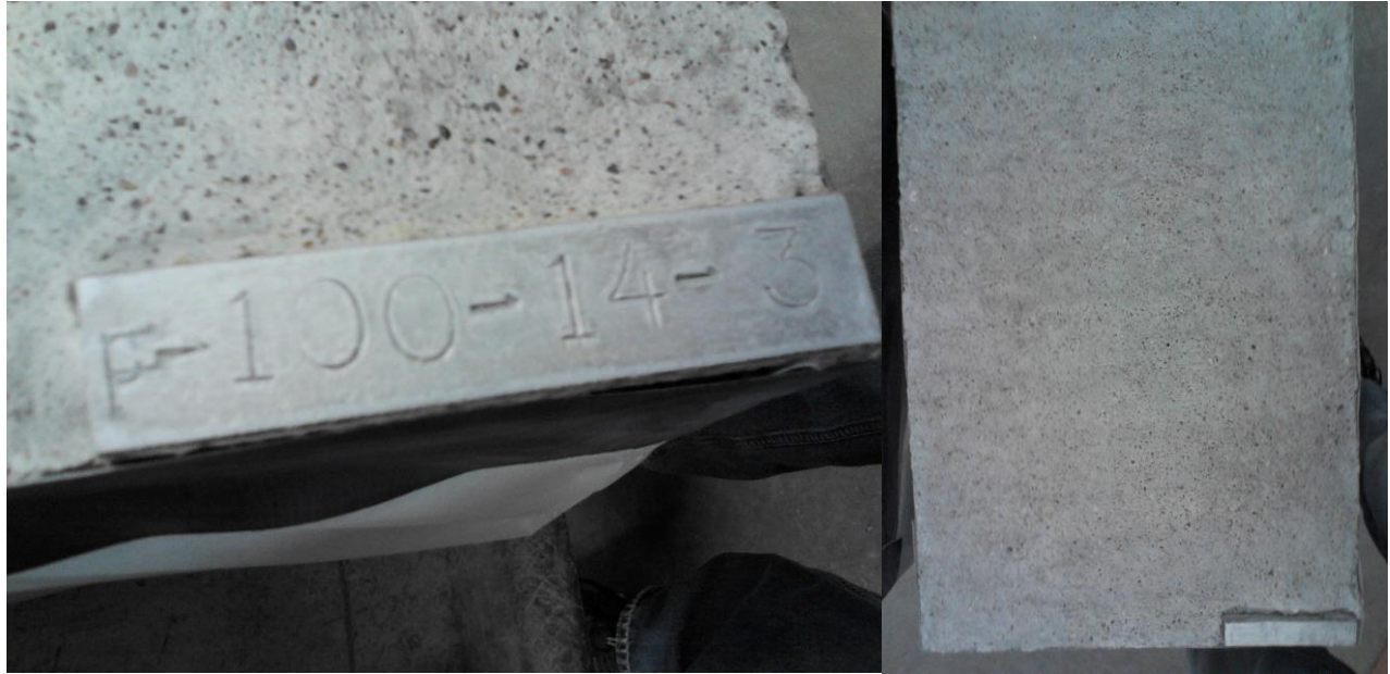
Figure 8: Slab label cast into the concrete
