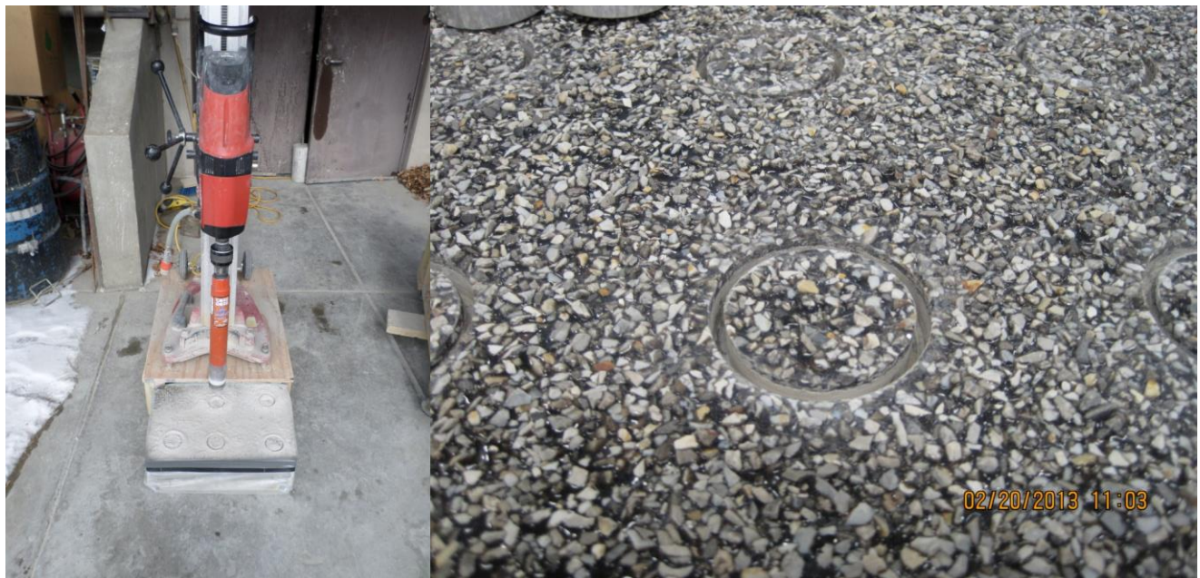
Figure 22: Coring setup (left) and a core through the overlay into the concrete (right).
