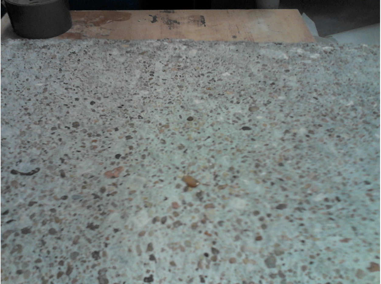
Figure 18: Close up of concrete surface after sand blasting
