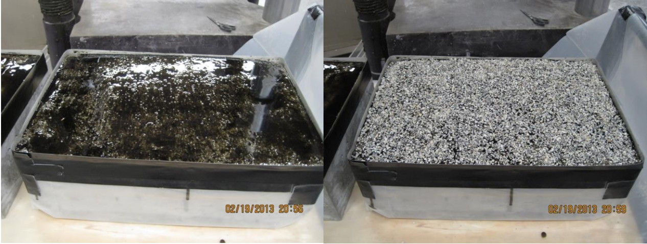
Figure 20: Placement of course 1 of epoxy (left) and aggregate (right)
