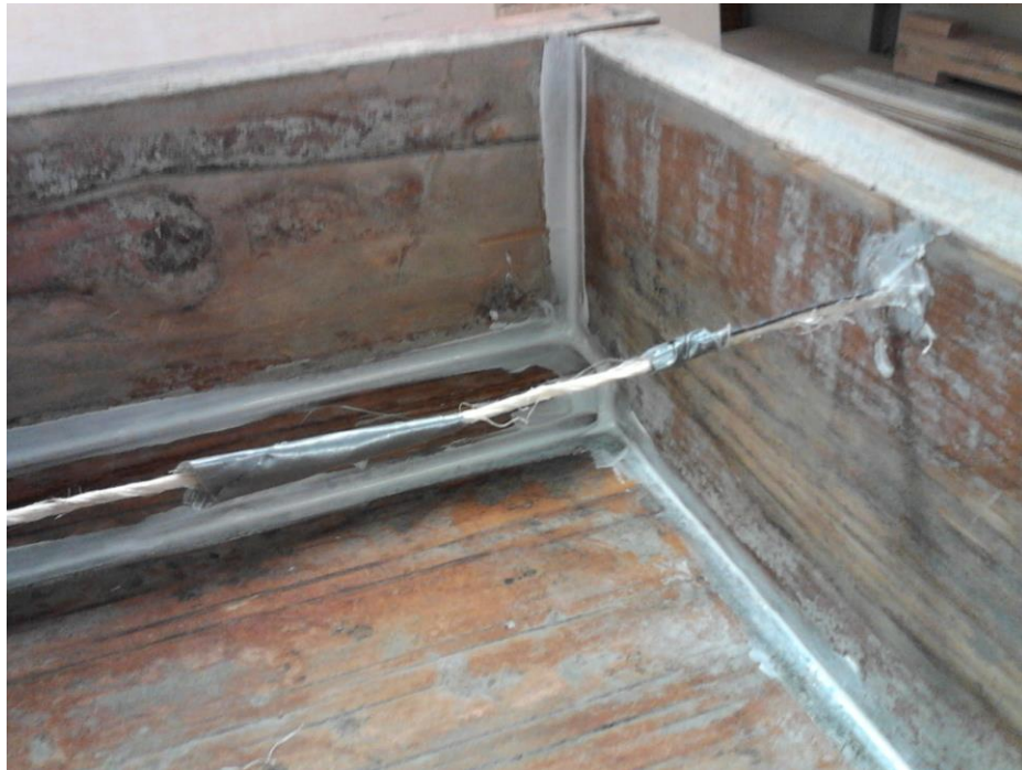
Figure 6: Thermocouple wire setup within slab forms
