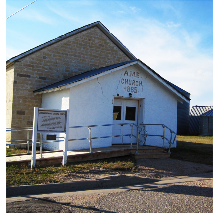
Figure 2.6: Site Visit: A.M.E. Church (by author, 2013).
