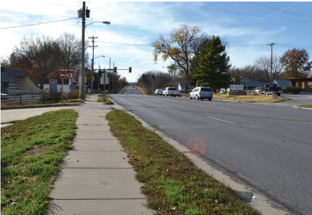
FIGURE 4.28 PRESENCE OF SIDEWALK ALONG ANDERSON AVENUE (HARPER, 2013).
