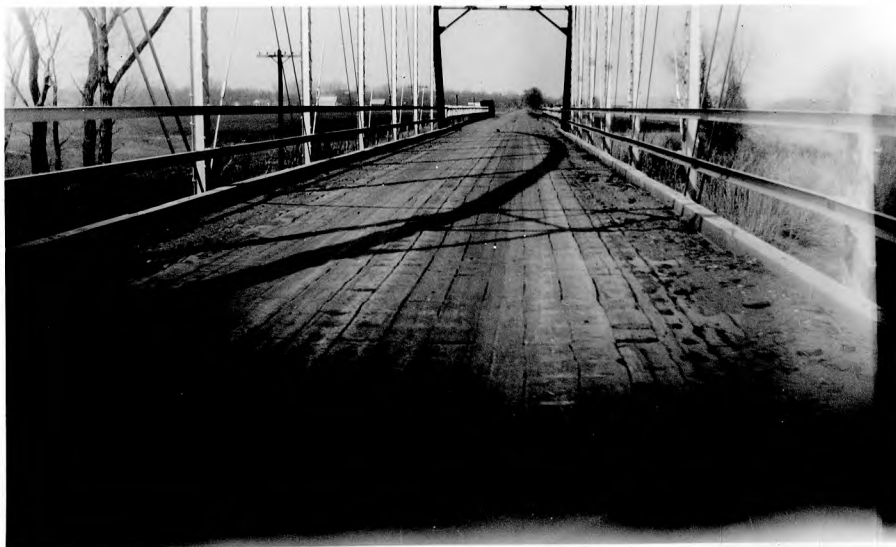
Fig. 3. Asphalt Plank Bridge Floor in Poor Condition.
