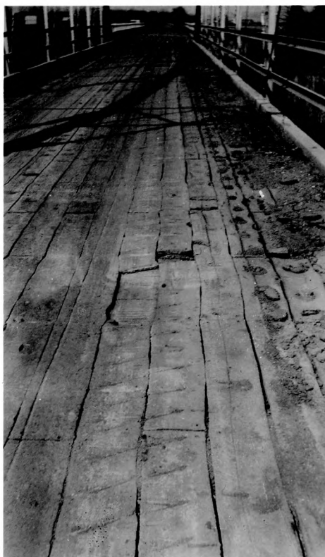
Fig. 4. Failure and Buckling of Asphalt Bridge Plank Floor.
