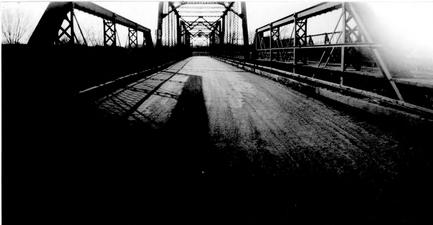
Fig. 7. Asphalt Bridge Floor Laid in 1928 in Excellent Condition.
