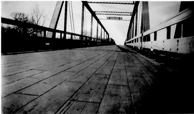
Fig. 8. Asphalt Plank Bridge Floor Showing Traffic Marks Indicating That the Planks are too Hard.
