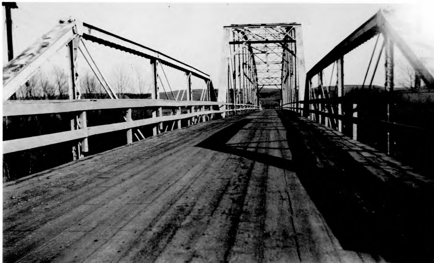
Fig. 6. Asphalt Plank Bridge Floor in Good Condition.
