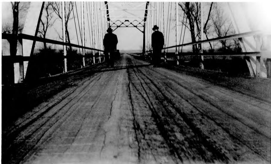
Fig. 5. Bridge Floor Laid in 1930 in Fair Condition.
