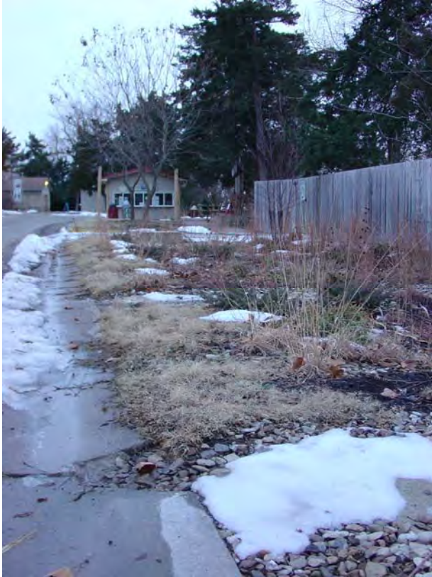
Cuts into the concrete gutter help move more water into the bio-retention garden while a soil moisture and temperature sensors assist Kansas State University faculty and staff to better understand the interrelationships between soils, vegetative growth, and climatic variables.
