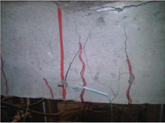
(a) Control Beam (B) at failure
