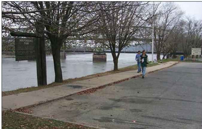
Figure 4- 40: Parking area prior to redevelopment where workers ate lunch and enjoyed the view (Atchinson Chamber of Commerce).
