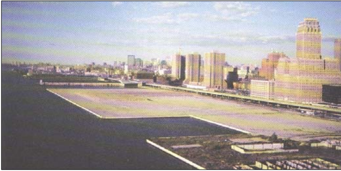
Figure 2-16: Battery Park site prior to construction (Breen, 1996).
