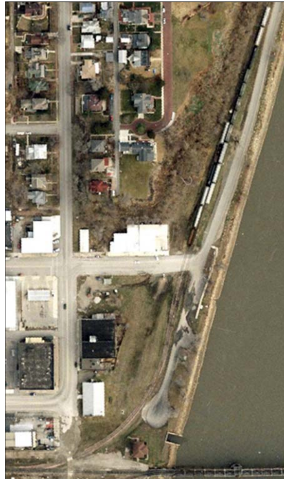
Figure 4- 41: Riverfront district prior to redevelopment (Atchinson Chamber of Commerce).
