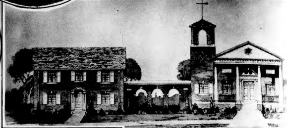
The new Methodist Episcopal Church and parsonage which is under construction in Millford, Kansas, by Dr. J. R. Brinkley personally, in memory of Doctor Brinkley's mother and aunt.
