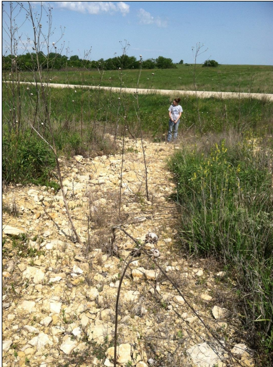
Figure 4.1. Rock fixed gully implemented to deter soil erosion at Fort Riley, KS
