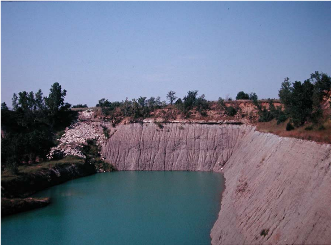
Figure 24. General view of the quarry exposure showing two walls or faces. Note the steepness of one of the walls that limits the access to the wall and makes it harder for a close observation.
