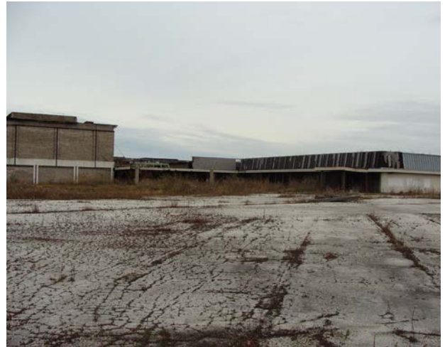
Above Figure 2.7 Dixie Square Mall
