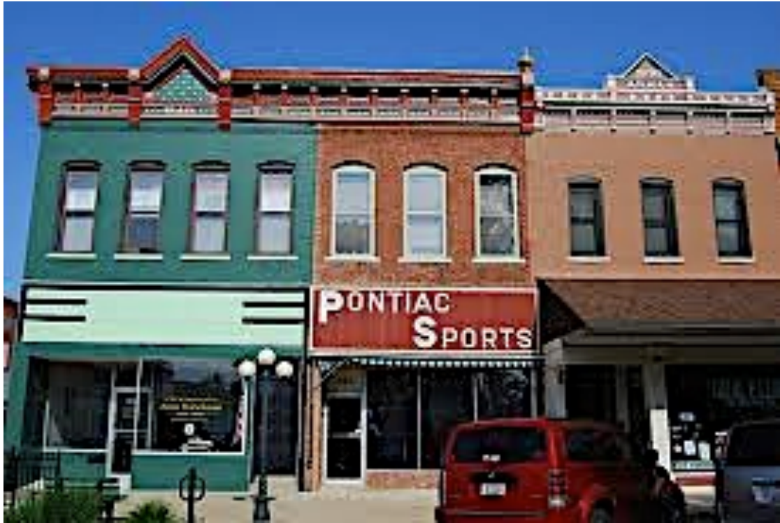
Figure 14: The reuse of brick to rebuild structures and maintain architectural style in Pontiac, Illinois (PROUD, 2010).
