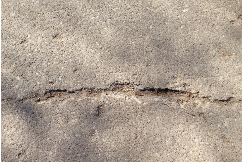
Figure 2.2 Spalling at transverse joint in concrete pavement
