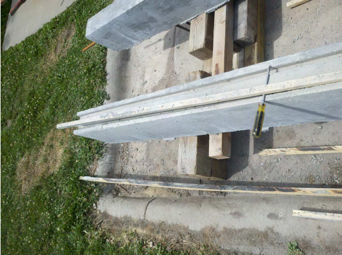
Figure 13: Chiseling out Wooden Pieces
