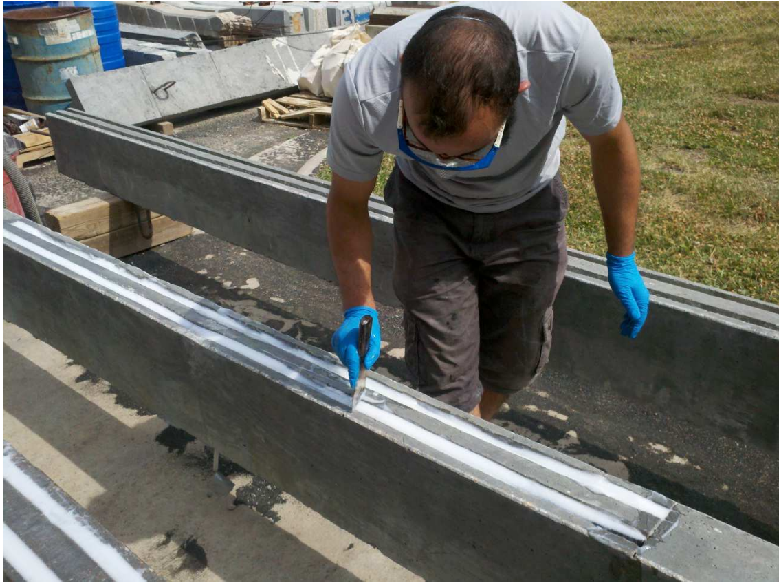
Figure 14: Scraping off Excess Epoxy during Installation of NSM bars
