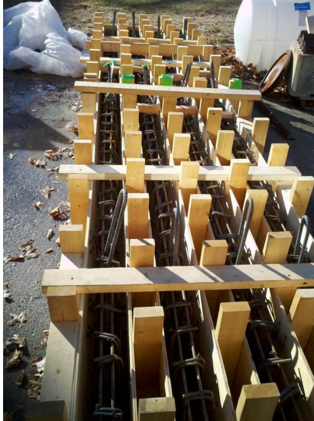
Figure 8: Steel Caging in Formwork before Casting
