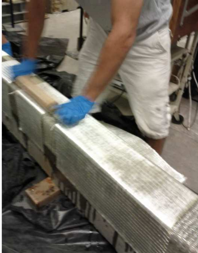
Figure 20: Removing Air Pockets by Rolling U-Wraps
