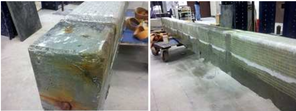
Figure 41: Corrosion from Salt (left) and Salt Residue (right)
