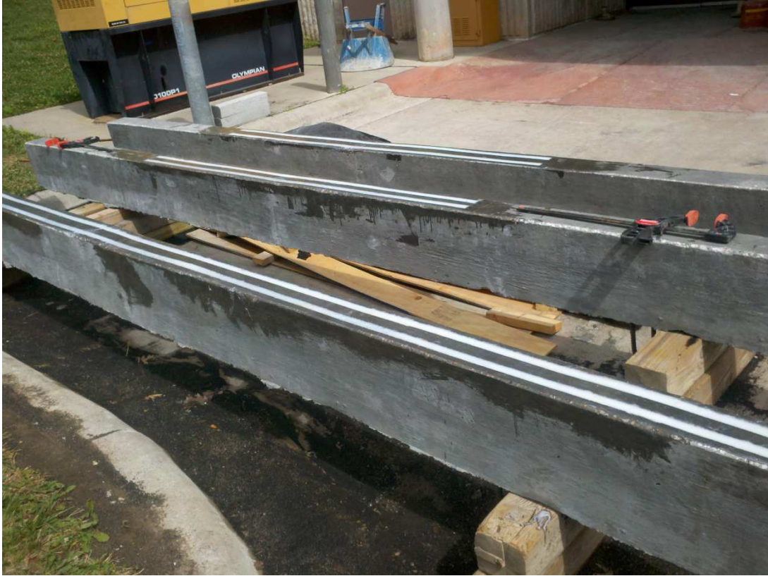
Figure 15: Beams with NSM bars Installed
