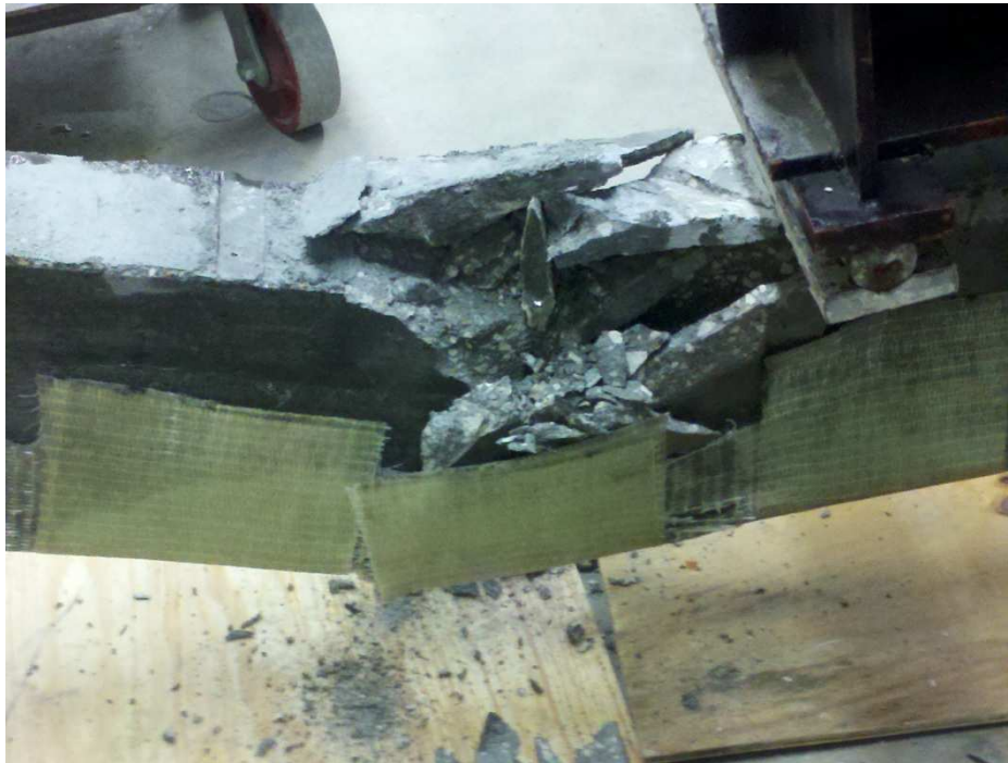
Figure 38: Failure of Beam R3
