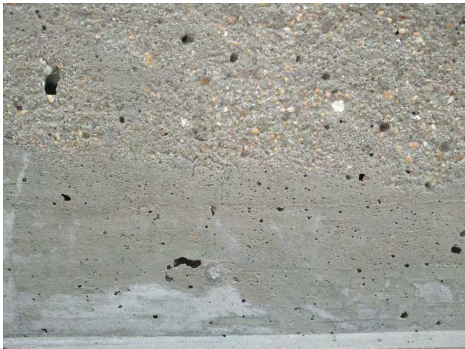
Figure 17: Comparison of Sandblasted (top) vs. Non-Sandblasted (bottom) Surfaces
