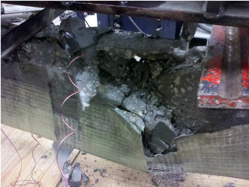
Figure 35: Concrete Crushing of Full Length NSM Beam
