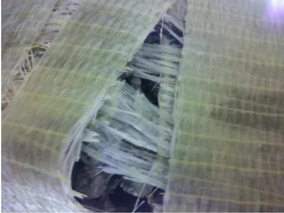
Figure 39: Rupture of GFRP sheet and U-wrap
