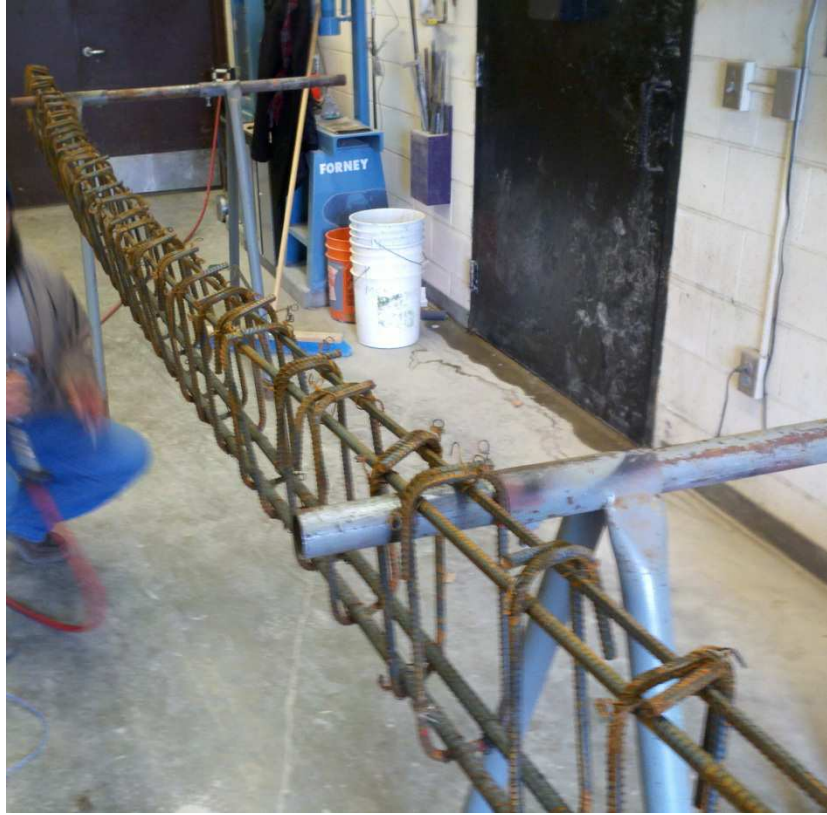
Figure 6: Steel Rebar Caging used for Beams
