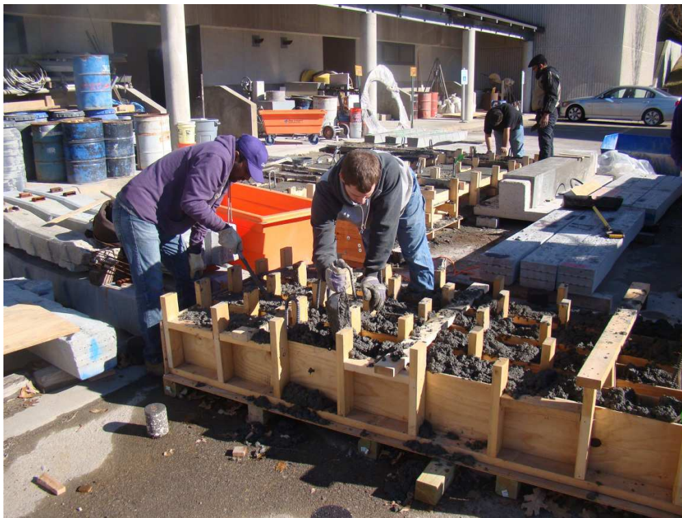
Figure 10: Casting of the Specimens
