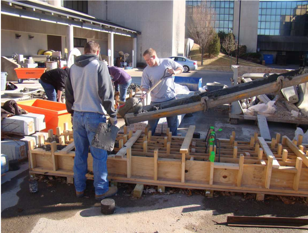
Figure 9: Casting of the Specimens
