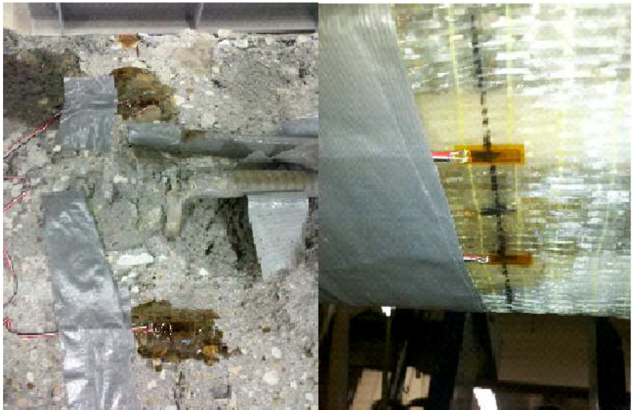
Figure 27: Strain Gages on the Concrete (left) and GFRP (right)
