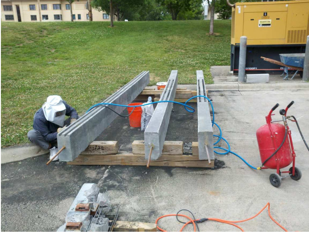
Figure 16: Sandblasting the Surface of the Beams
