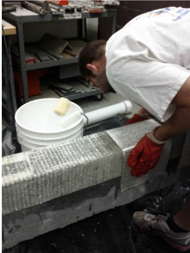
Figure 19: Applying U-Wraps
