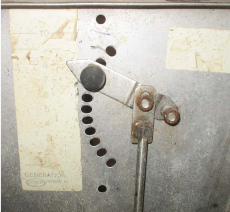
Figure 4.1 STACO stainless steel dry feeder on feeder setting 3
