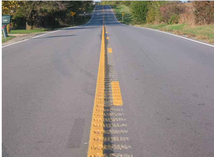
(Milled Centerline Rumble Strips)
