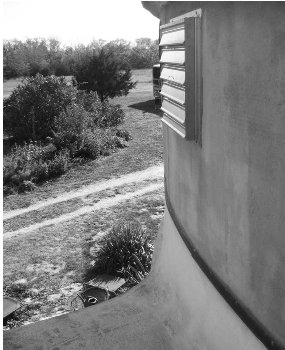
View from Roof
