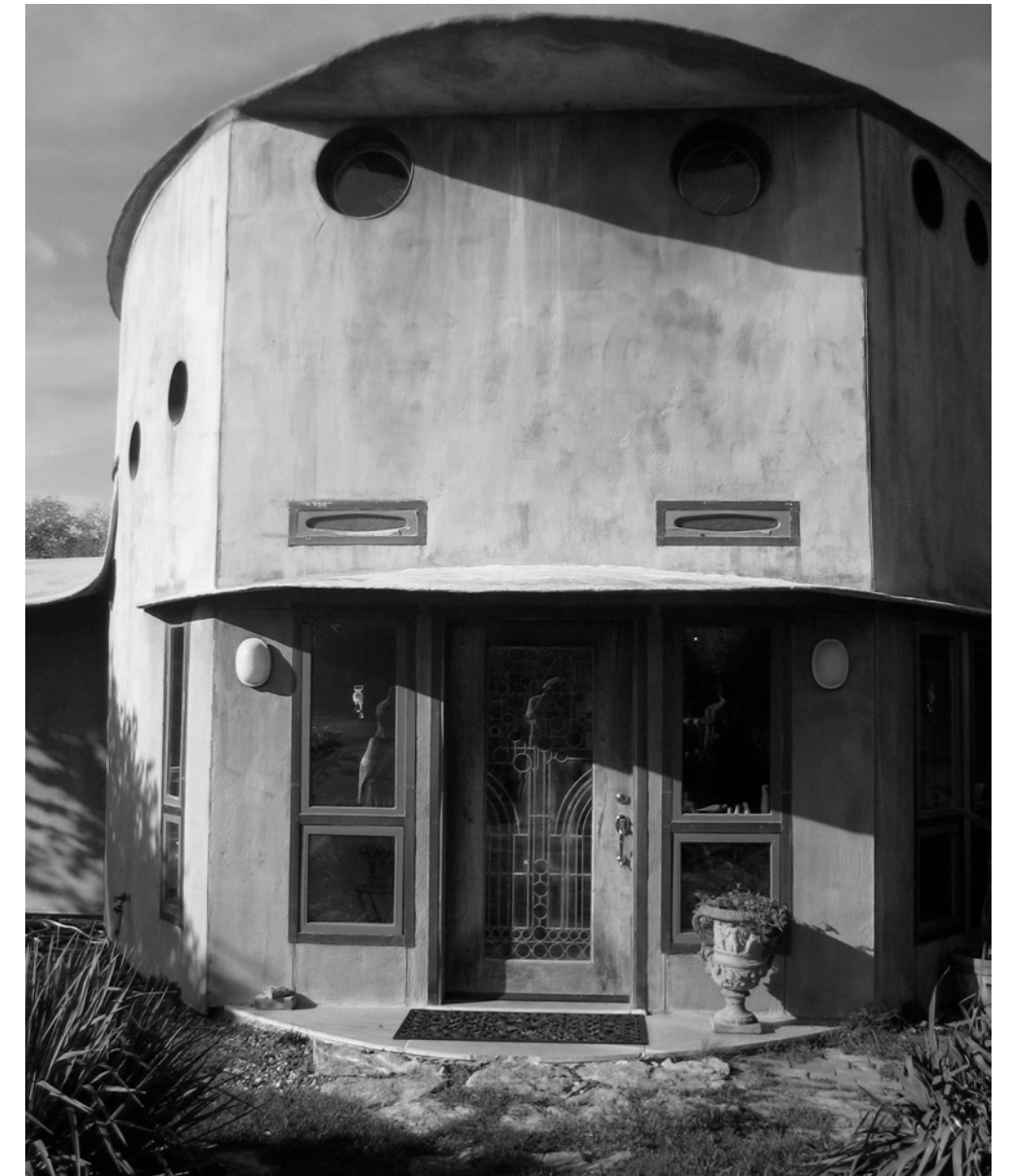
Entry at Southern Facade
