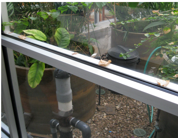
Fig. 2. The 'Living Machine' inside the Anita B. Gorman Discovery Center, used to treat all waste water (Kingery-Page)
