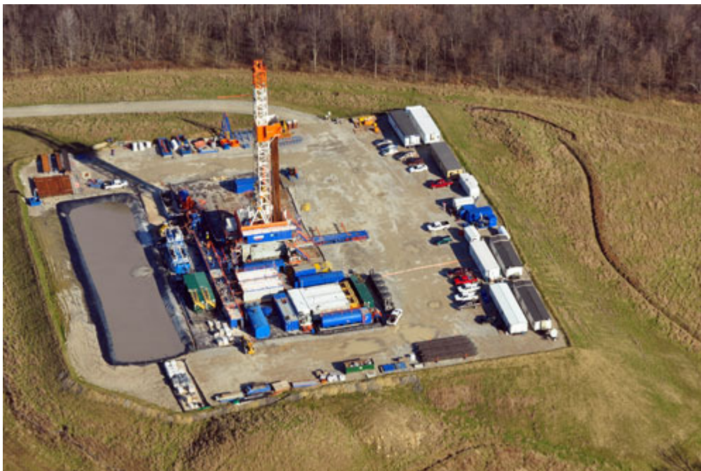
Figure 1.1 Photograph of a typical fracturing and drill pad 5
