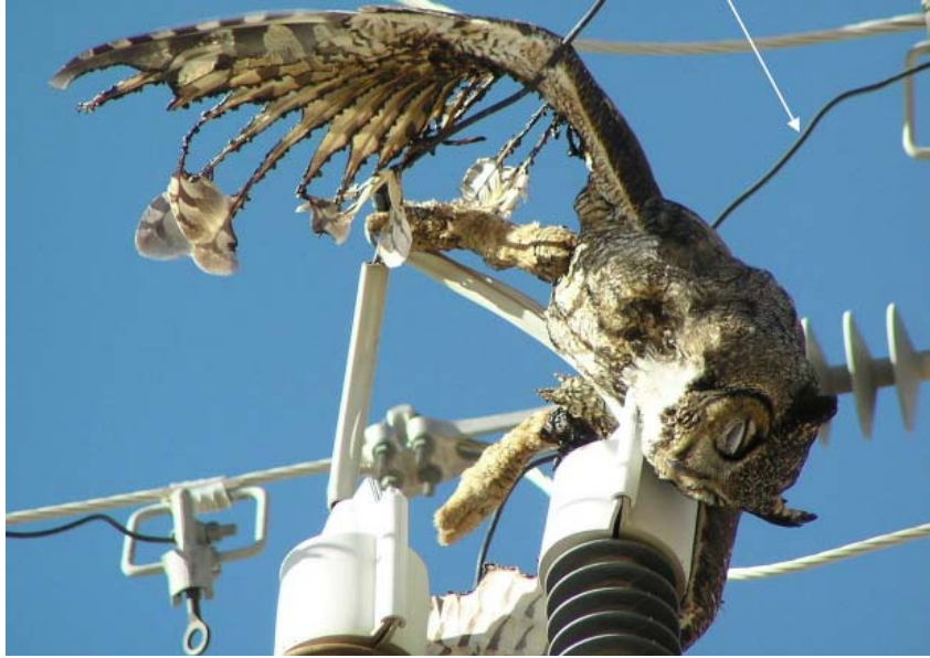
Figure 1.1 An Owl Caused Outage in the Distribution System [75] (With Permission of Rick Harness)
