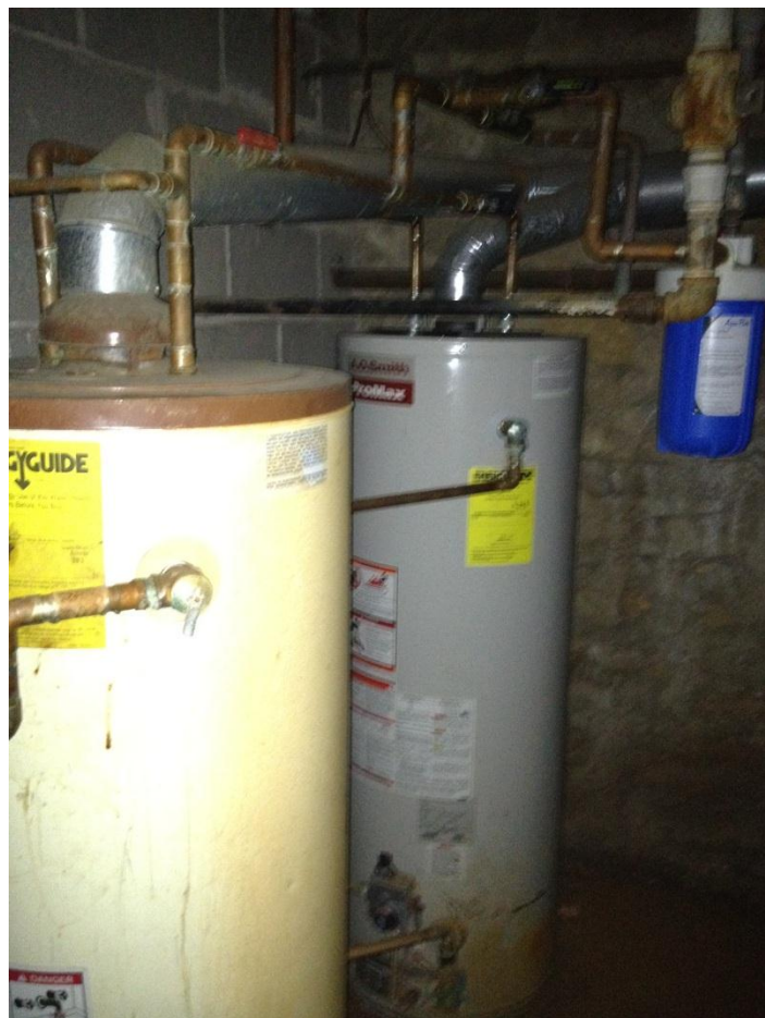
Figure A-12 Water Heaters
