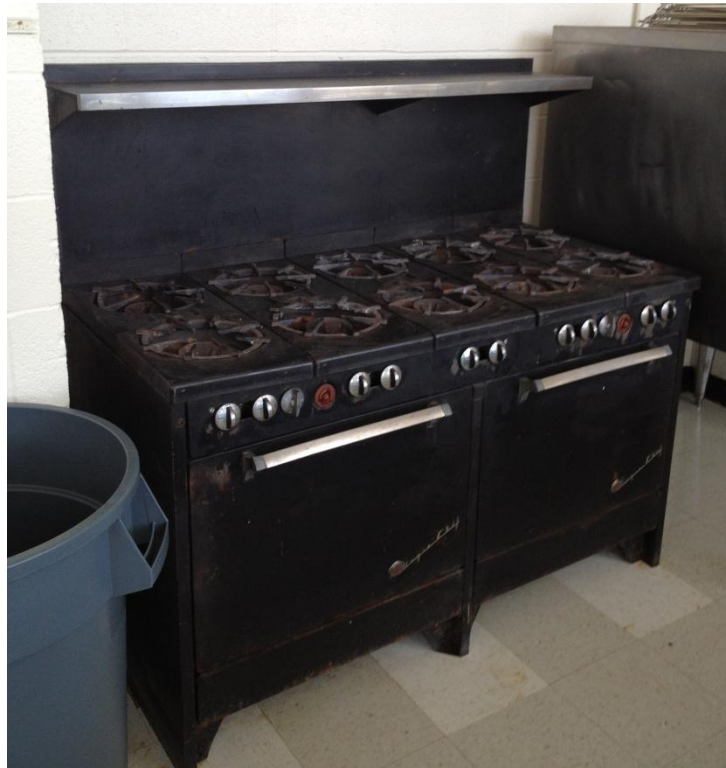
Figure A-22 Kitchen Stove with Hood
