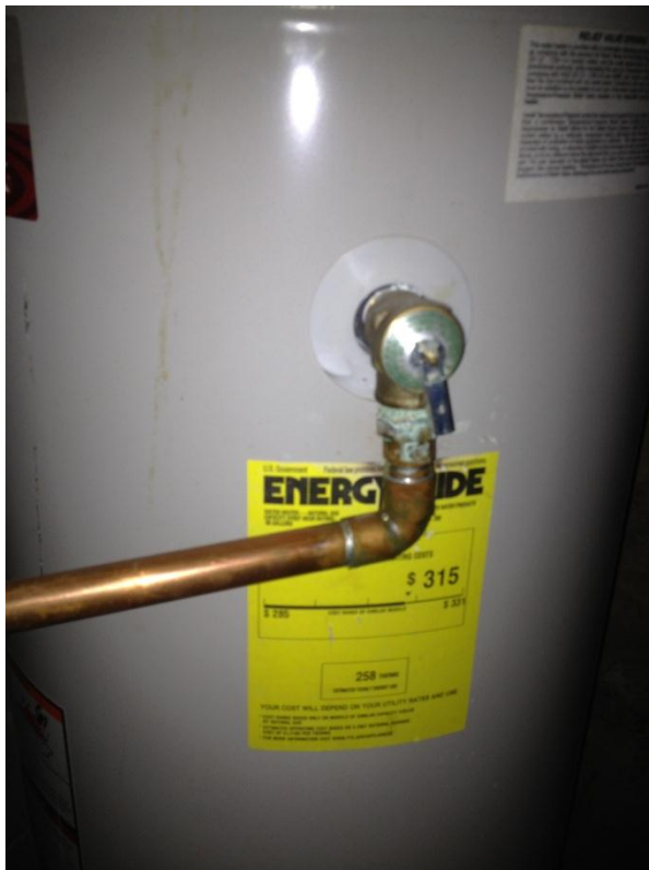
Figure A-16 Water Heater 2 Energy Star Label
