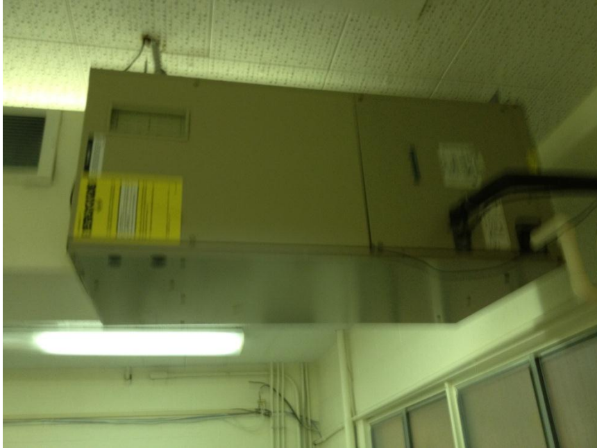
Figure A-18 Fan Coil Unit in Office Area Near Kitchen
