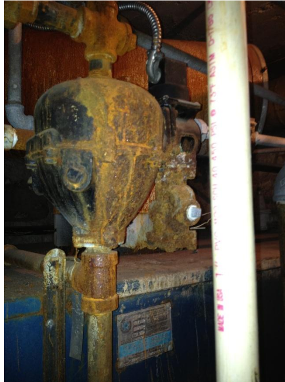
Figure A-9 Boiler 1 Degradation
