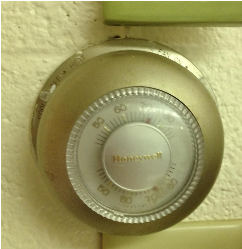
Figure A-20 Fan Coil Thermostat
