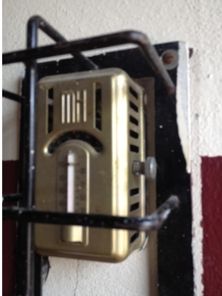
Figure A-29 Gymnasium Temperature Sensor
