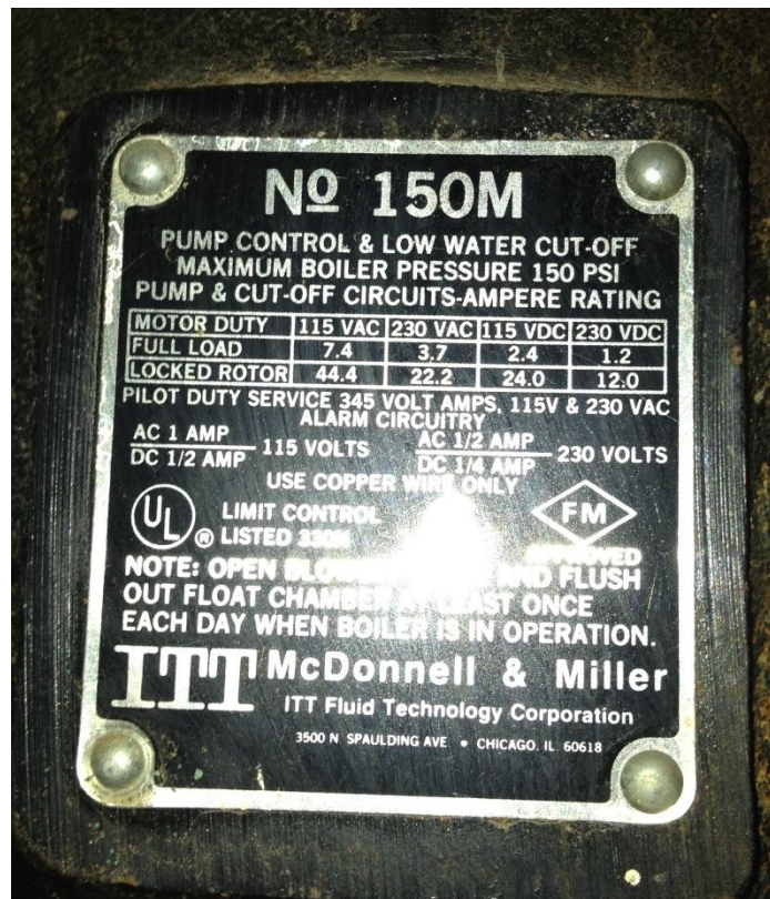
Figure A-10 Boiler Pump Name Plate
