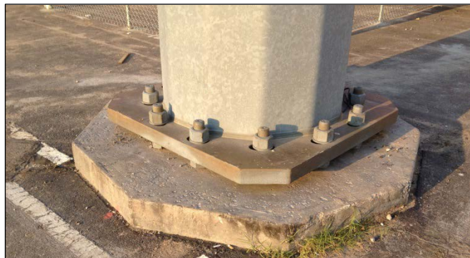
Figure 1 - Stadium Light Pole Attachment
