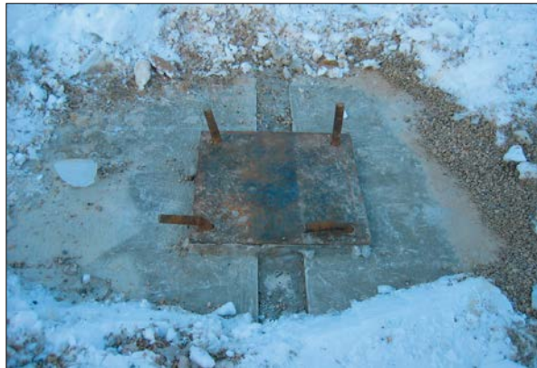
Figure 15 - Bent Anchor Rods (AISC DG1, 2010)
