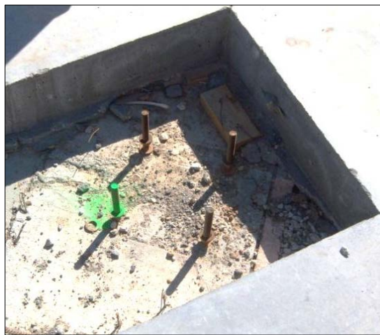
Figure 3 – Cast-In-Place Anchor Group
