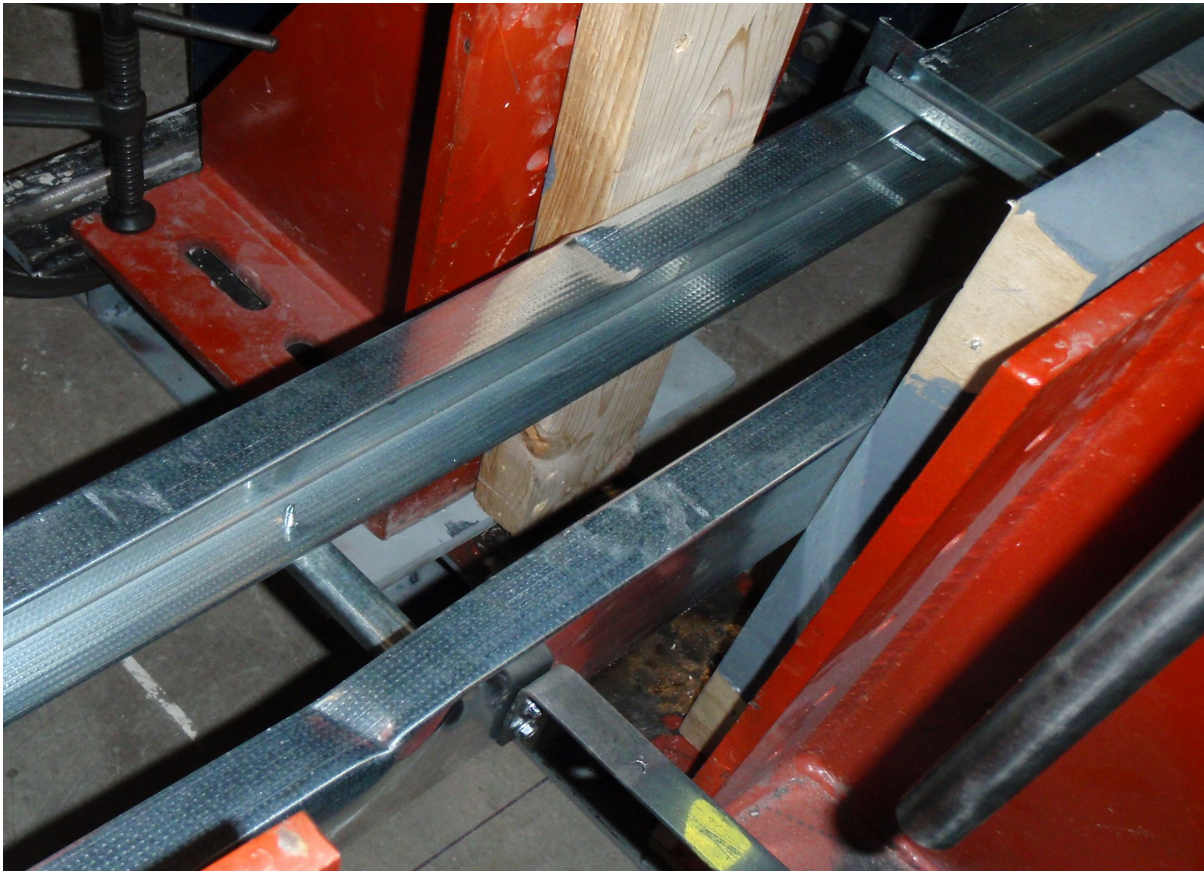
Figure 3.1: Typical Failure in a 3 \frac{5}{8} " beam.
