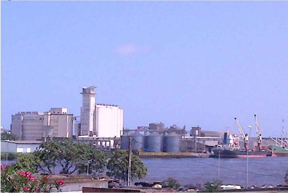
Figure 1.3: General view of GMA silos and flour mill
