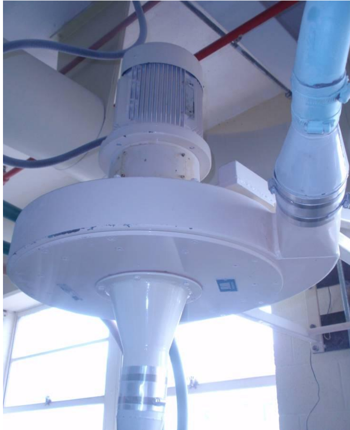
Fig.2.16 Robinson Impact Detacher (Henry Simon Robinson Inc., Stockport, UK).
