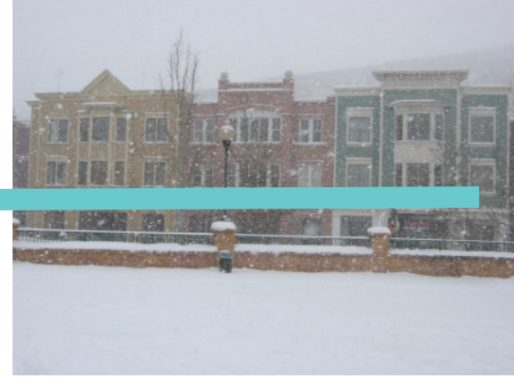
Figure 2.54 Facades (Cody Peratt 2008)
