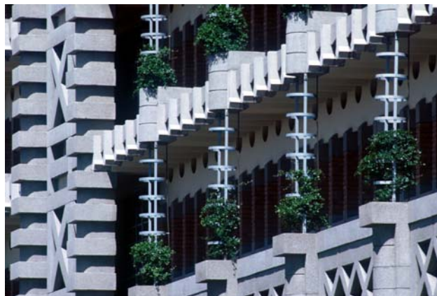
Figure 9. Eastgate's masonry and concrete exterior walls inspired by the 900-year-old walls of Great Zimbabwe. Photograph copyright 1997 Michael Pearce Partnership/Aga Khan Trust for Culture, used with permission. Retrieved February 5, 2009 from http://archnet.org/library/images/one-image.jsp?location_id=3167&image_id=36901 .
