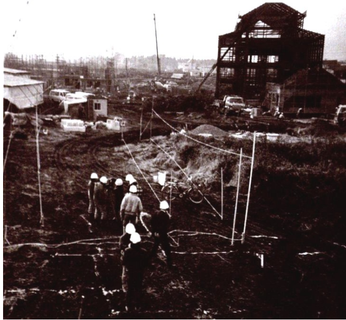
Figure 21. On-site staking and flagging design process to determine the approach towards the main gate from the first gate on the Eishin campus. Photograph copyright 1985 Center for Environmental Structure, used with permission.
