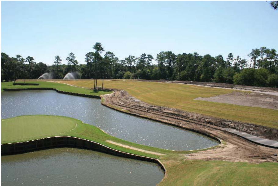
Figure 2.3 - Sodding 18th Fairway of TPC Sawgrass ( Maccurach Golf Construction, 2003 )
