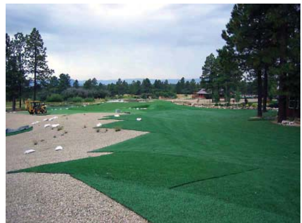
Figure 3.3 -Echo Basin Ranch partial synthetic turf installation (Echo Basin Ranch 2005)
