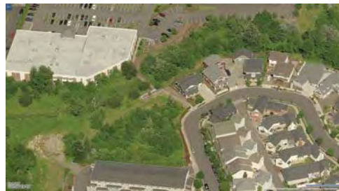
Fig. 3-16 Pedestrian bridge over stream (Virtual Earth 2008)
