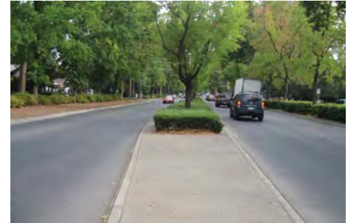
Fig. 3-27 Esplanade Center Median
