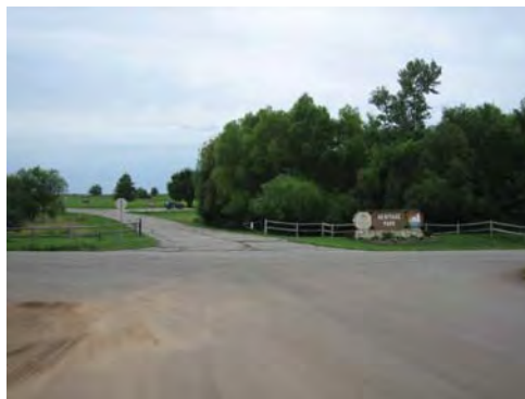
Fig. 2-108 173rd Street crossing Pflumm and entering Heritage Park
