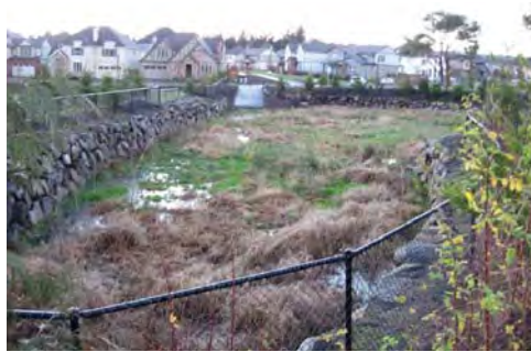
Fig. 3-100 Large Retention Pond
