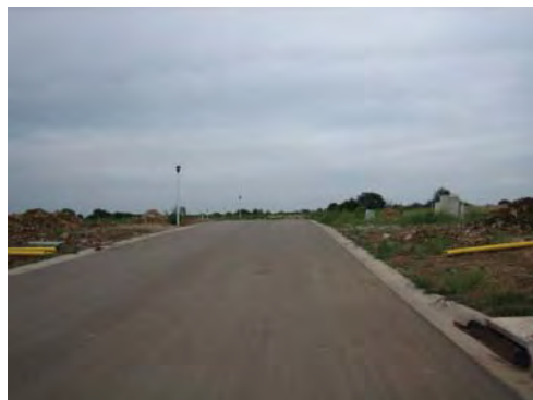
Fig. 2-107 173rd Street in Chapel Hill Subdivision Photos: David Vogel 2008
