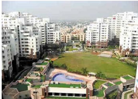
Figure 2.5: View of new apartment complexes in Kolkata today
