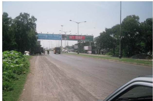
Figure 2.21: View towards the Kasba Junction
