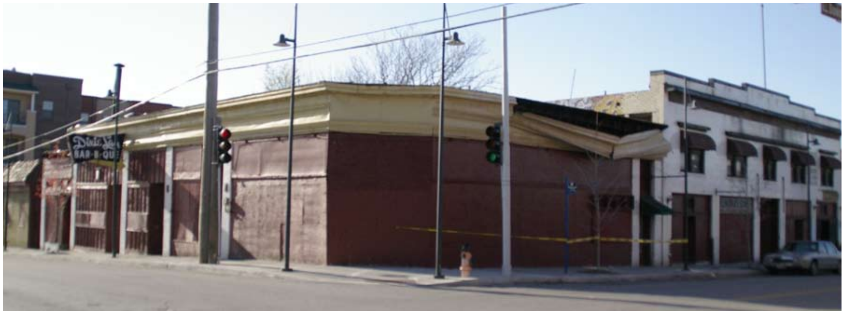
Figure 4.32: 19th and Vine: Historical Image (Kansas City Star 1929)- Present Photo: Deterioration (taken by author)
