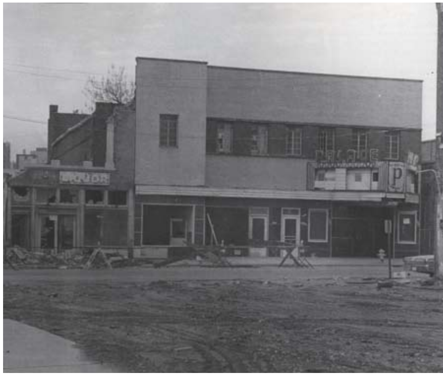
Figure 3.6: Destruction of Palace Theater (Worley 1998)
