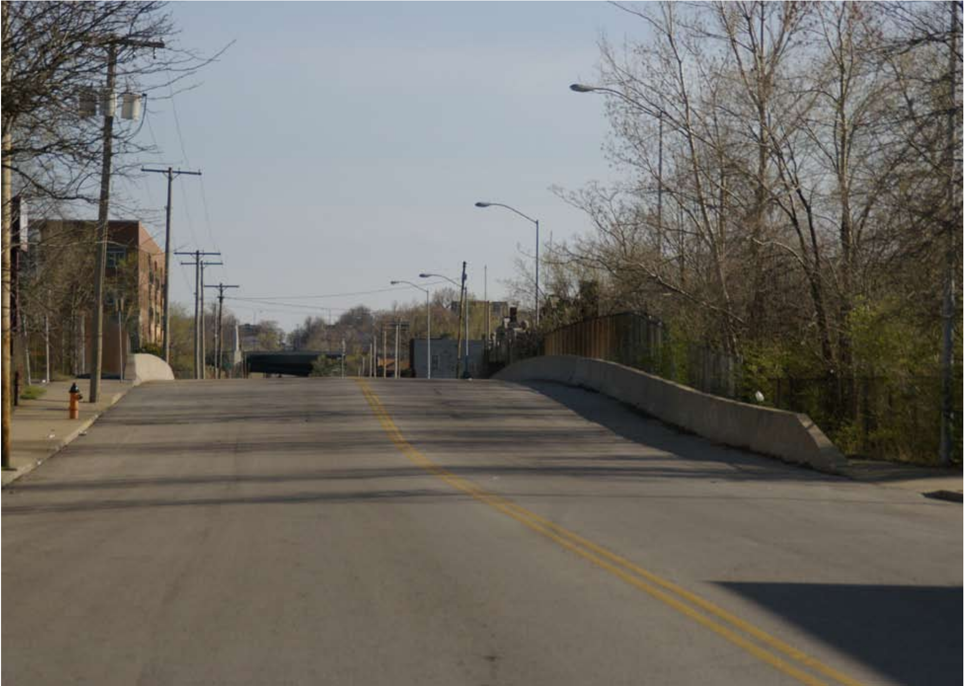
Figure 4.35: Pedestrian Connection across railroad tracks on Vine Street (taken by author)
