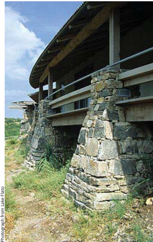
Figure 6.6 Native Stone Piers
