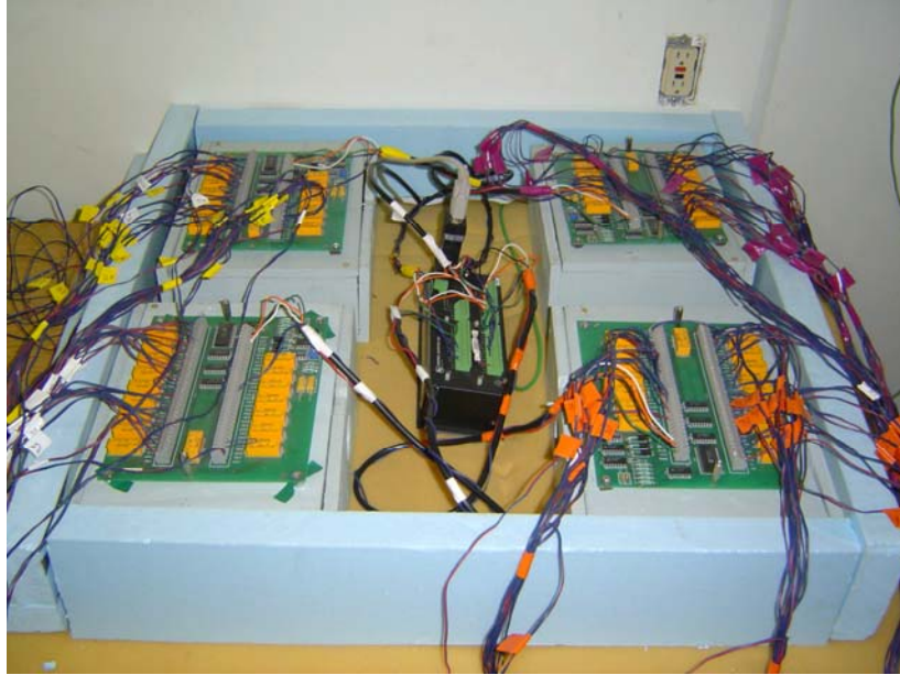
Figure B.5 The datalogger (center) and four multiplexers with thermocouples connected.
