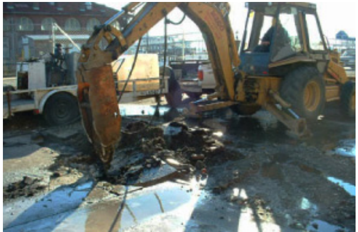
Figure B.39. Breaking Pavement.
