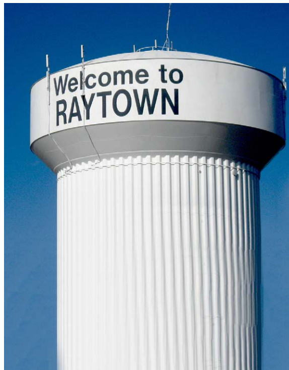
Figure 4.10. Active 2-million Gallon Water Tower In CBD. Pumphrey 2012.
