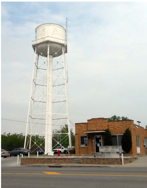
Figure 4.9. Inactive Water Tower at Headquarters. Pumphrey 2012.
