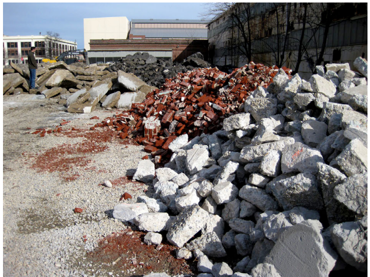
Figure B.40. Sorting and Stockpiling Salvaged Materials.
