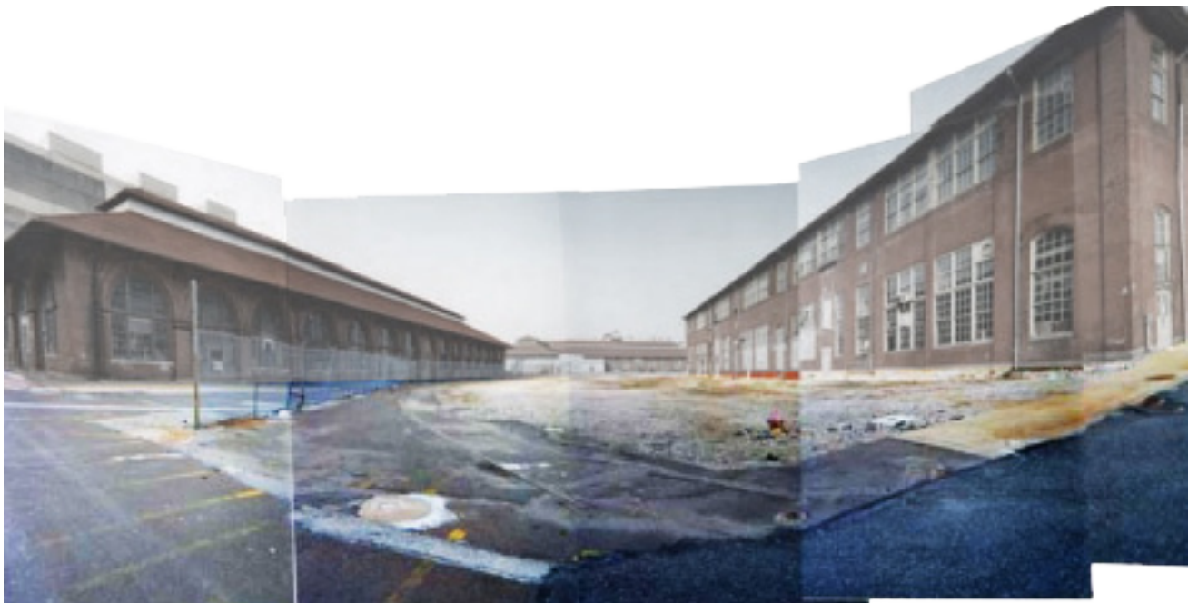
Figure B.34. Asphalt and Concrete Covered Site. Color Adjustment by Pumphrey 2011. Source: Bargmann 2011, 61.
