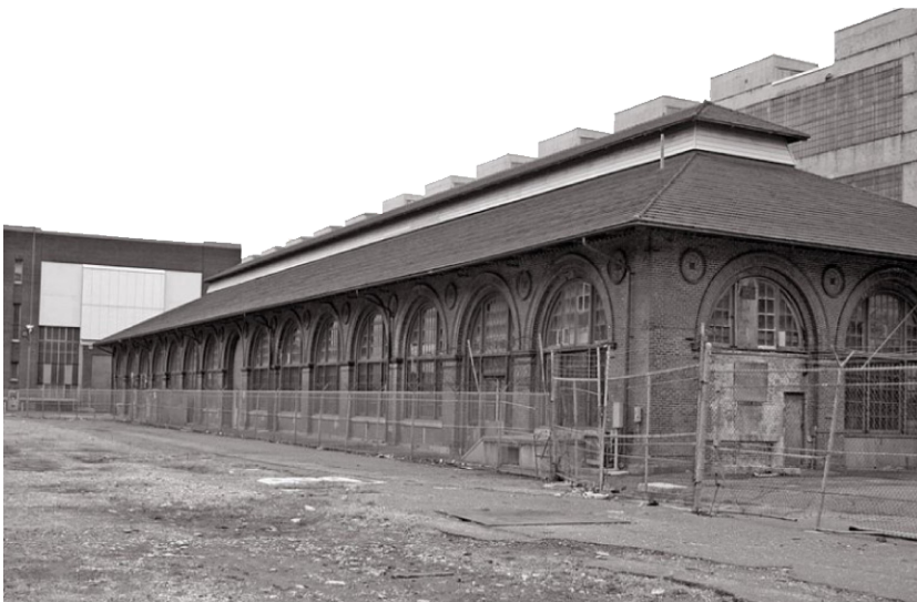
Figure B.33. Dilapidated Buildings. Source: MS&R 2005.
