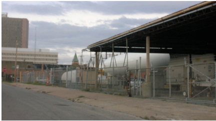
Figure 1-6: Above Ground Storage Tanks (taken by author)
