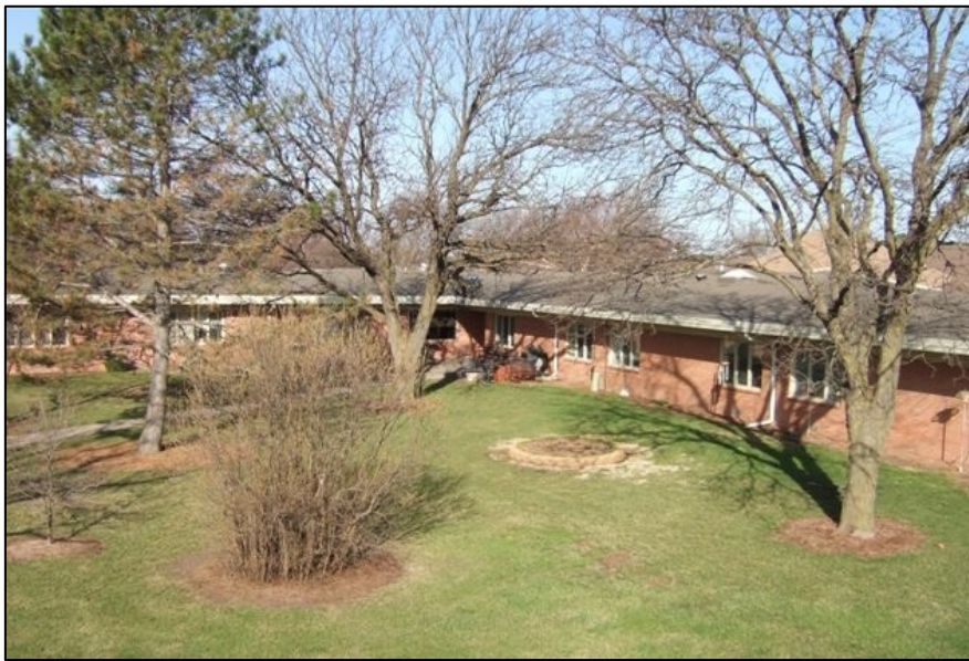
Figure 3.3 Existing Schowalter Courtyard, Northeast Corner, April, 2010.
