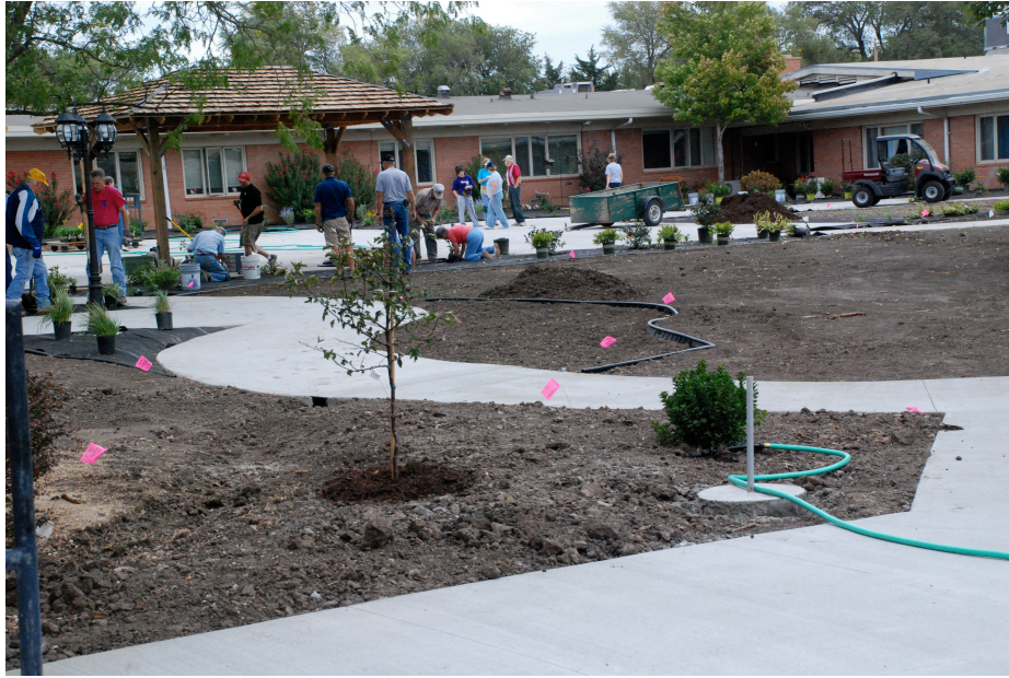
Figure B.9 Schowalter Courtyard, October, 2011, From Maintenance Access Looking Northeast.
