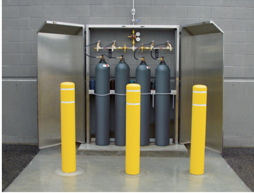
Figure 3-4 Hydrogen Storage Tanks Located Outdoors [E]
