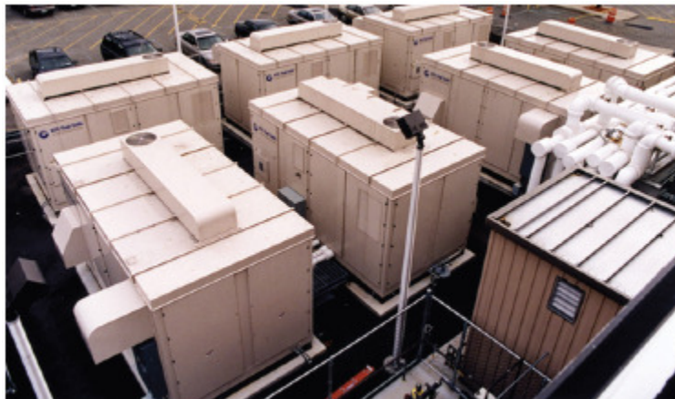
Figure 5-3 UTC Power's PureCell Model 200 Fuel Cells at Verizon Call Routing Center [M]
