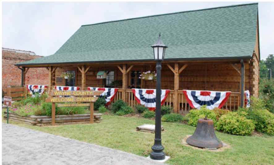
Figure 6: Welcome Center, Collinwood, TN (Natchez Trace Reservation Services, n.d.) Additional photos, see Appendix C.
