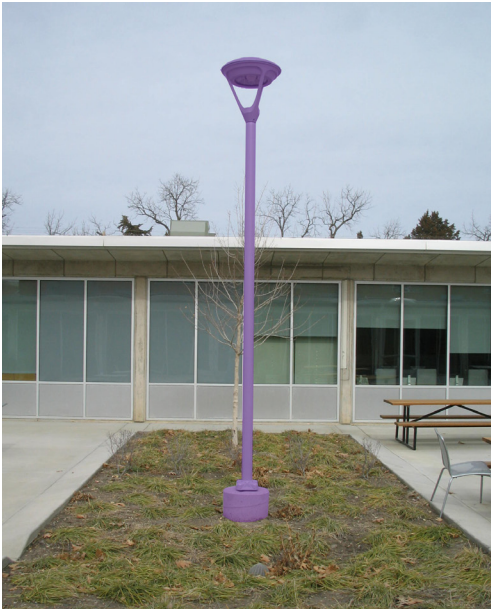
Lack of sufficient exterior lighting
