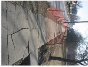
Cracking sidewalk adjacent to Blair Park.
