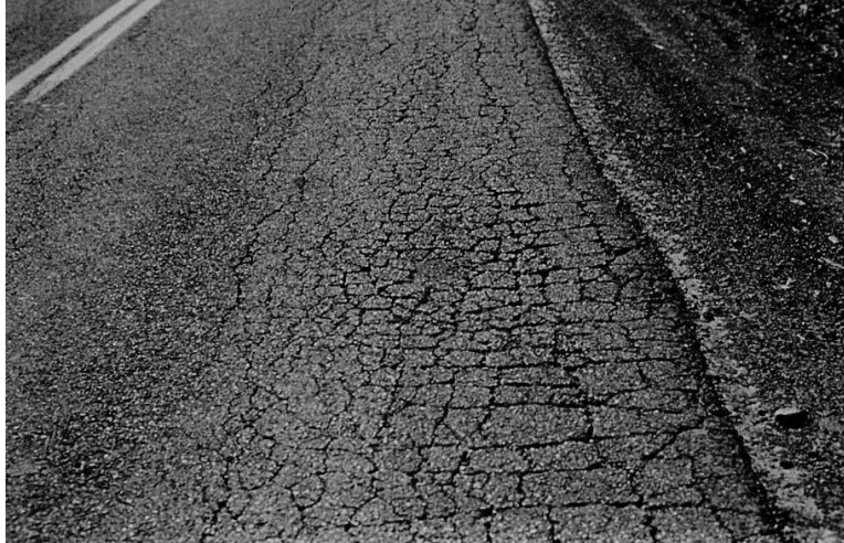
Figure 2.3: Example of Fatigue Cracking
