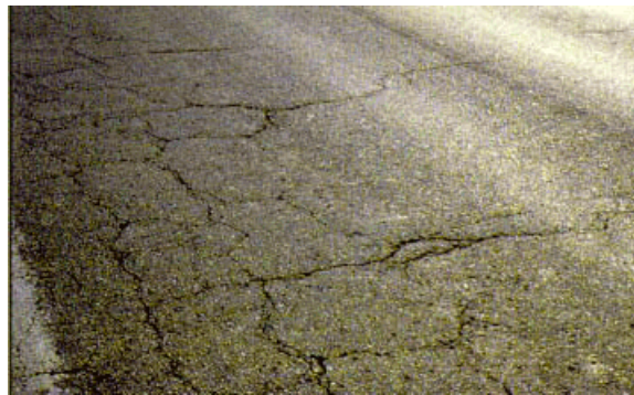
Figure 2.2: Example of Block Cracking
