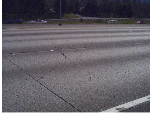
Figure 2.4: Example of a Corner Break
