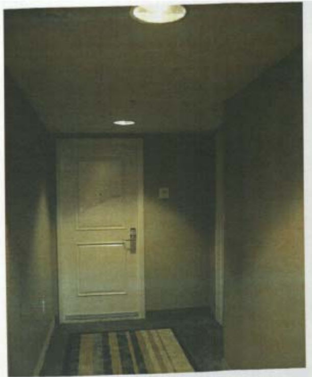
Figure 41. The scalloped light patterns (shown) on hallway walls should be avoided. Luminaire light distributions should be selected to light walls evenly. This is particularly important in corridors where visitors need to find apartment numbers and residents need to see faces clearly through doorway peepholes. (photographer: Eunice Noell-Waggoner)
