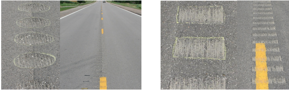
Figure 1.9 Patterns of Milled-in CLRS installed in Kansas
