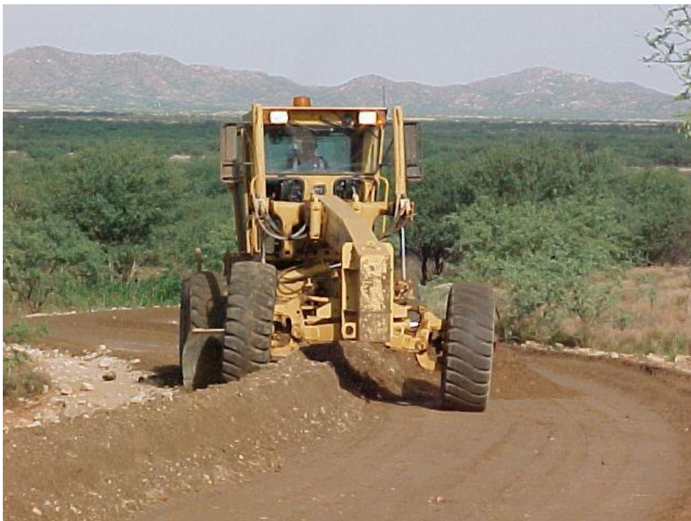
Figure 2-3: Blending of borrow material with lignin product [source: Surdahl et al , 2005]
