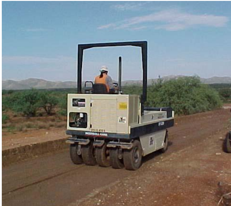
Figure 2-4: Rolling and compaction of blended material surface [source: Surdahl et al. , 2005].
