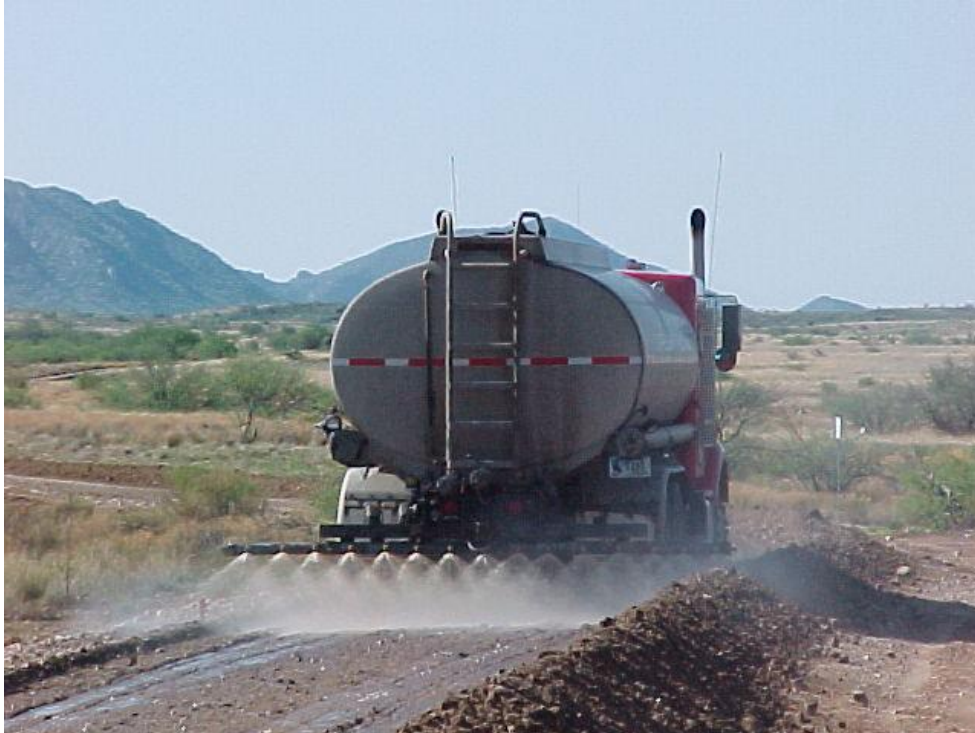
Figure 2-2: Spray application of Lignin product to bladed surface [source: Surdahl et al , 2005].
