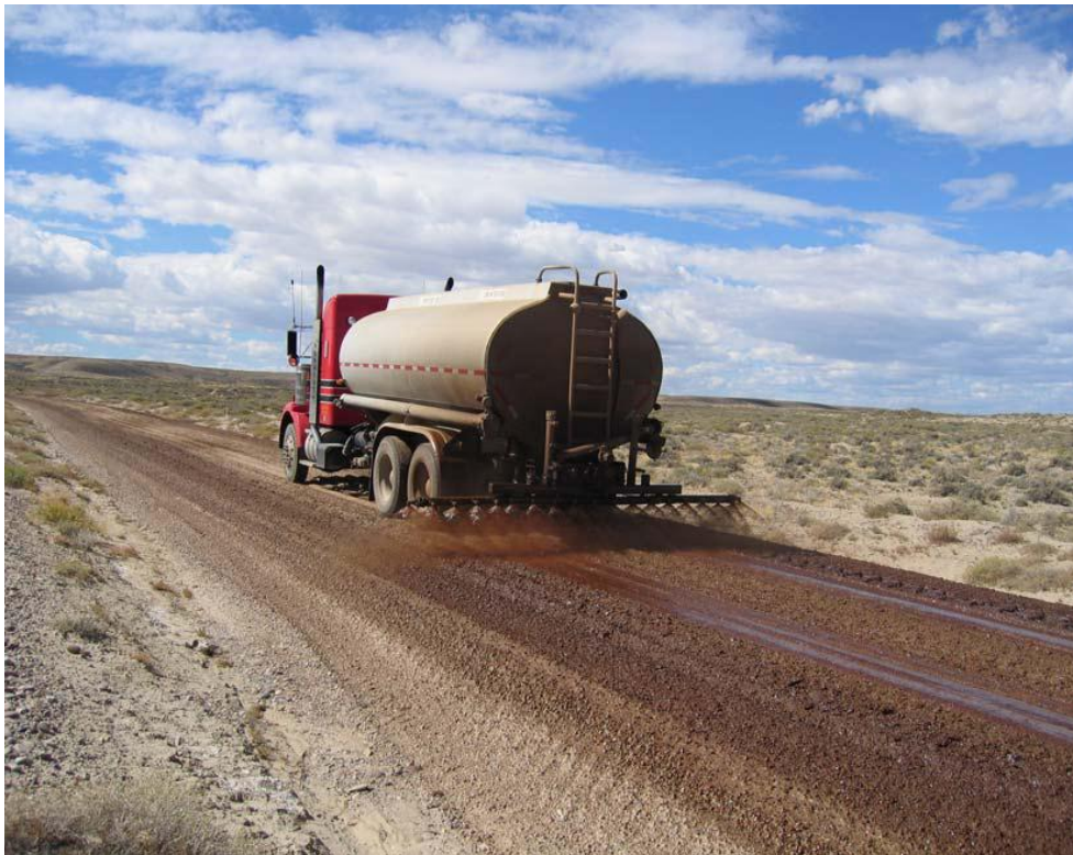
Figure 2-5: Application of Lignin-based product at Seedskaadee National Wildlife Refuge [source: Surdahl et al , 2008].
