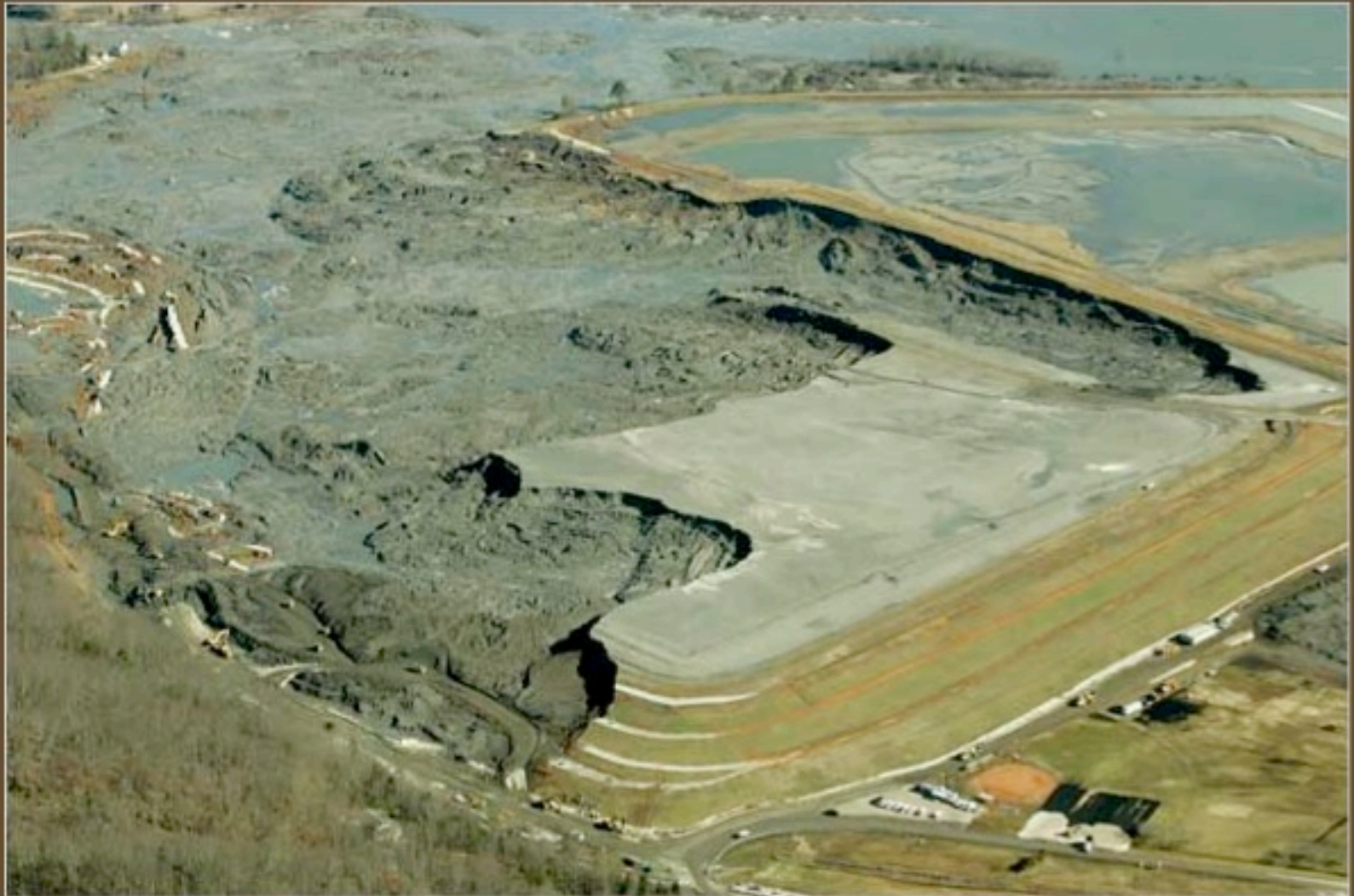
The 40-acre pond, whose dam broke, was used by the Tennessee Valley Authority as a containment area for ash generated by the coal-burning Kingston Fossil Plant in Harriman, Tennessee
