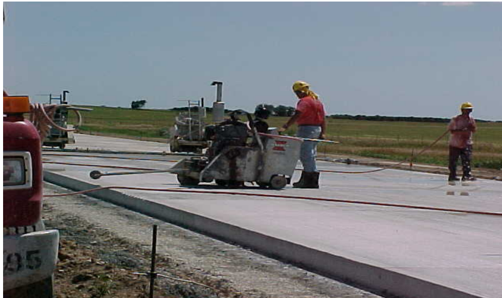
Figure 2.9 Typical joint sawing operation in Kansas
