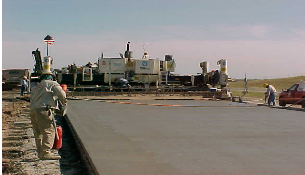
Figure 2.8 PCCP paving operation in Kansas
