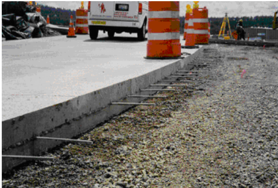
Figure 2.7 Deformed tie bars
