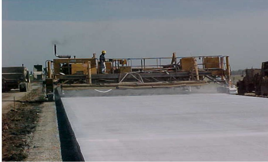
Figure 2.10 Curing operation using liquid membrane forming curing compound
