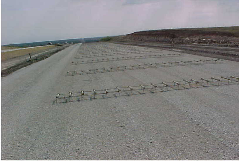
Figure 2.6 Typical dowel layout
