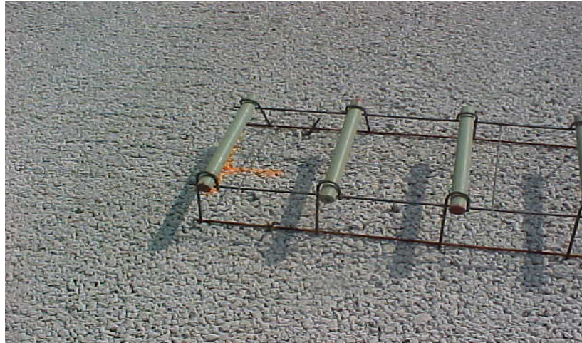
Figure 2.5 Short steel dowel bars
