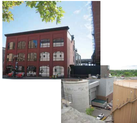
Figure 4.5 Energy District power plant
