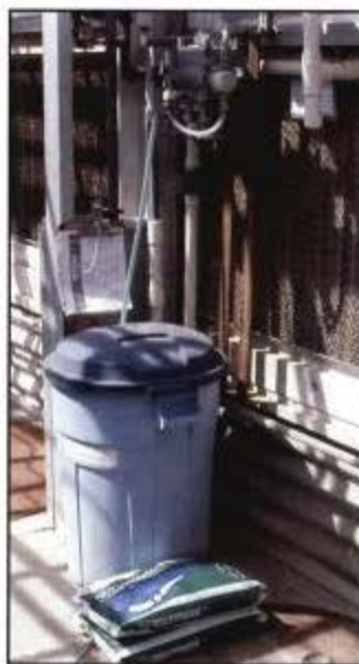
Figure 6-5. Fertilizer used through this Smith injector is easy to track if, each time a bag is mixed into the stock tank, it is recorded on the clipboard hanging nearby. (Photo by Marci Spaw, Kansas State University)
