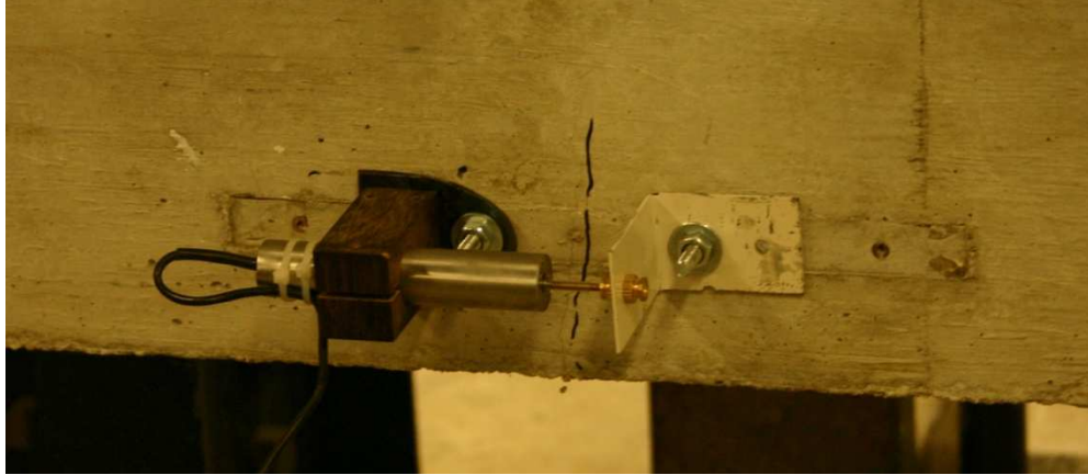
Figure 6.3 LVDT mounted to measure crack width
