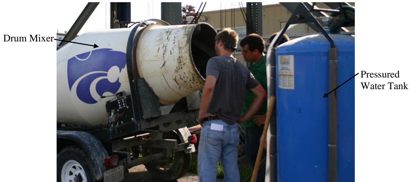
Figure 3.8 Adding Water to Mixer
