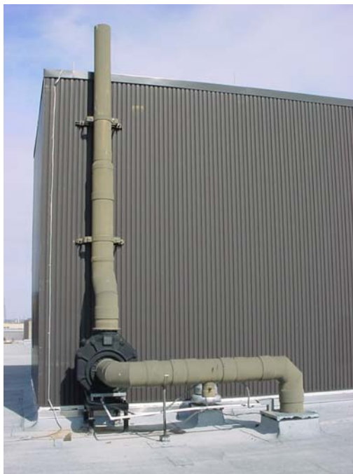
Figure 3.1.2 Ammonia Chamber Exhaust Vent on Roof of Rathbone Hall
