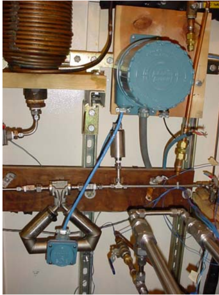
Figure 3.2.15 Ammonia Flow Loop Flow Meter
