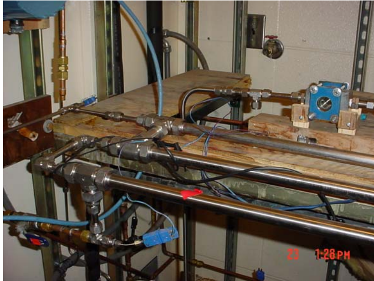
Figure 3.2.7 Ammonia Flow Loop Conditioner
