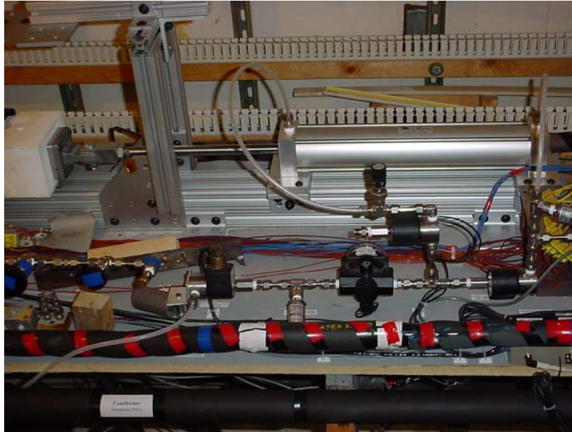
Figure 3.3.1 Picture of Raytheon Test Cell Pneumatic System
